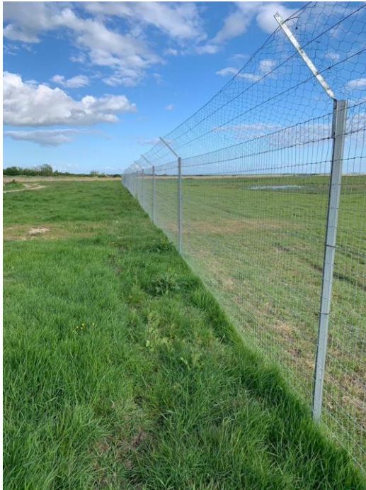
Figure 3-1. Example of a fox proof fence installation. Note that the vegetation along the outside edge (left hand side of the photo) has fully recovered following replacement over the buried skirt.
